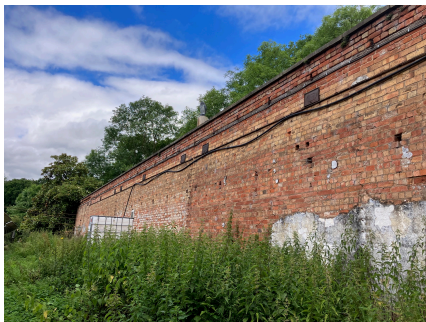
North wall showing brickwork, coping and heating vents
