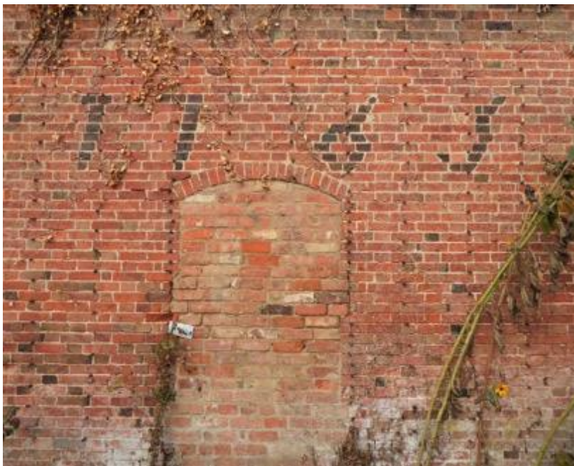
WKG East Wall with date, 1765, & blocked entry
