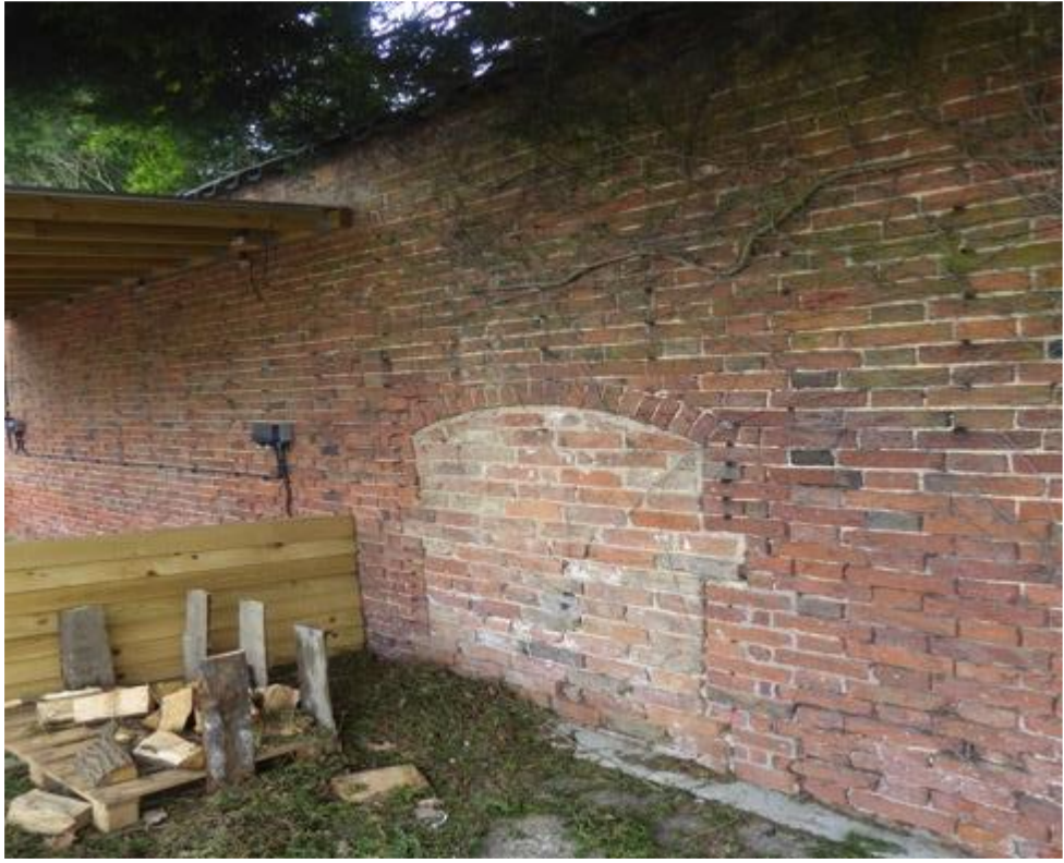
WKG West Wall with blocked entry
