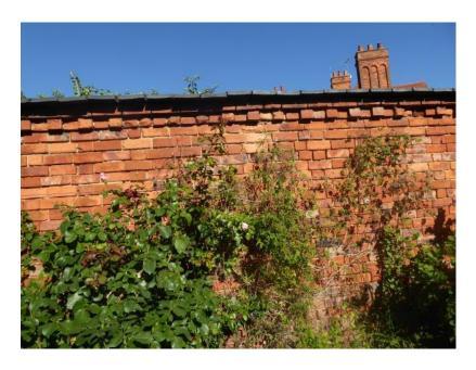
Original NE Wall of the WKG at Westbrooke House showing the brick bond, cornice and coping.
