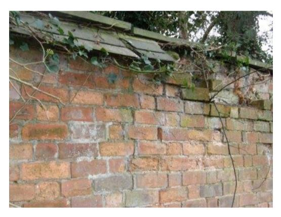
This is the outside of the north wall of section 1. This shows the double slate drip course.
