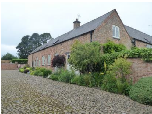
6. The converted stables and coach house forming the west wall of Saddington Hall WKG.
