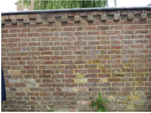
4. Close-up of the east end of the original street wall of Saddington Hall WKG with billet patterned brickwork beneath coping.
