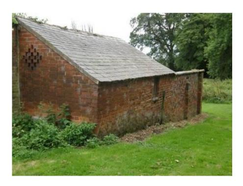
Lean-to shed taken from the outside of the WKG, situated against the southern end of the west wall. On the near wall is the diamond shaped section of brickwork for ventilation. The wall at the far end of the shed projects beyond the South wall of the WKG as it is now
