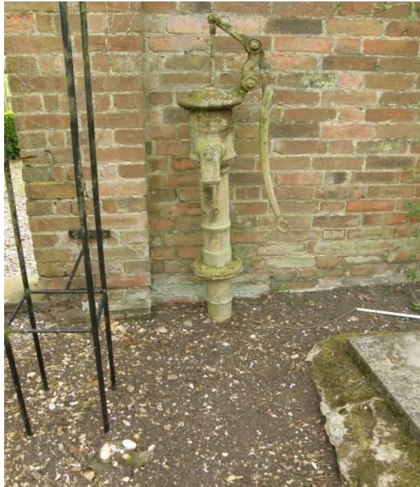
Pump outside wooden gate in north wall over old soft water tank
