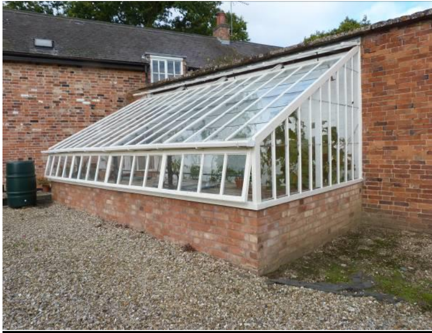
1927/8 Messenger greenhouse in N/W corner
