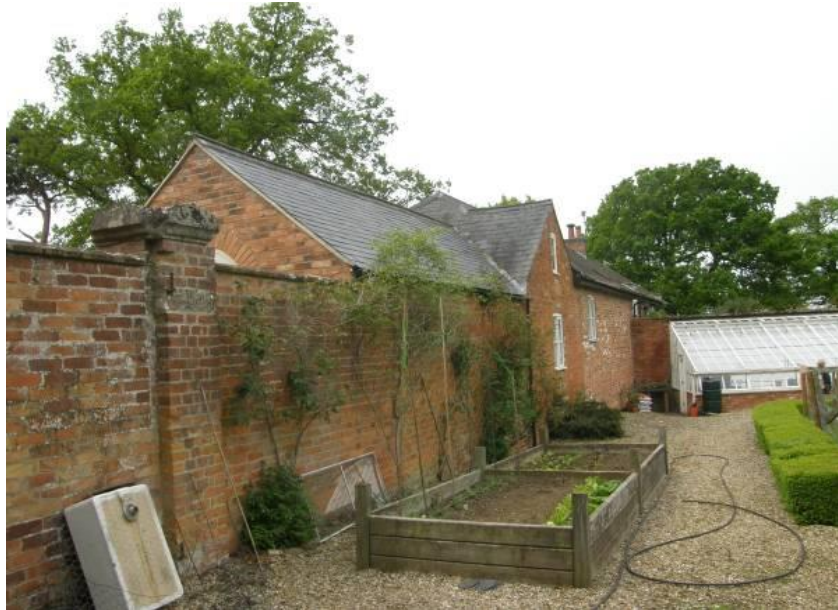
View of west side of walled garden showing raised beds on the foundations of original cold frames and greenhouse. The bricked up wall into the old farmyard can be seen on the left.
