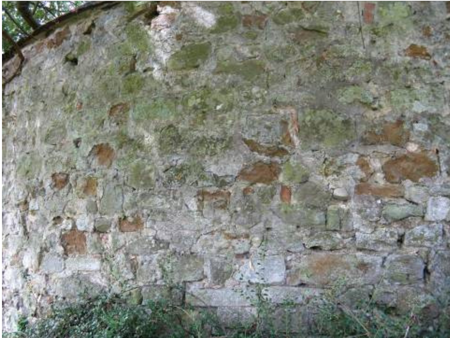
Remains of original wall, showing stonework and coping
