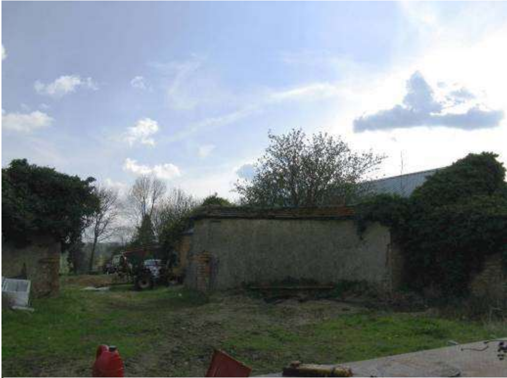
Remains of entrance forecourt walls, looking south
