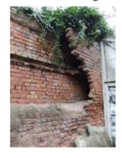
example of a heated wall. As it is partly derelict, it is possible to see the brickwork of the ducting that carried the heat round the walls.
