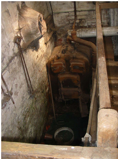
Left: Ideal Standard Boiler (Photograph Sue Blaxland September 2006)
