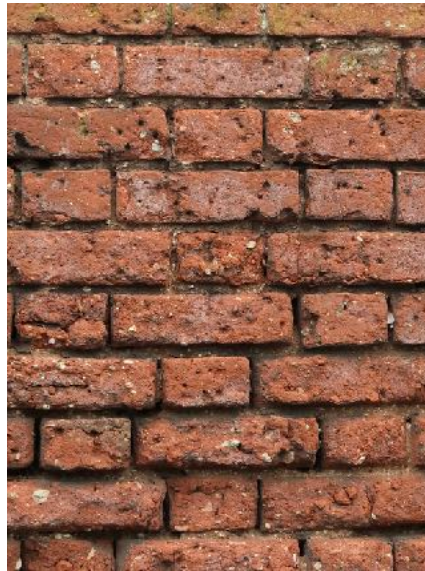
Figure 8: Close up of brick wall at Whatton House Walled Kitchen Garden showing Flemish bond. 28th August 2018. (Photo: Sheila Burnage)
