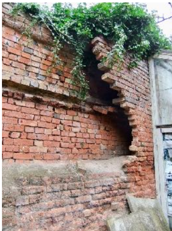
Figure 9: View of part dismantled hot wall, revealing how it was constructed. Whatton House Walled Kitchen Garden north wall. 28th August 2018. (Photo: Sheila Burnage)
