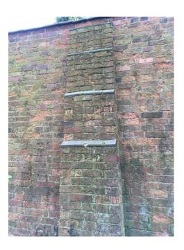
Exterior of north wall, showing stepped buttresses
