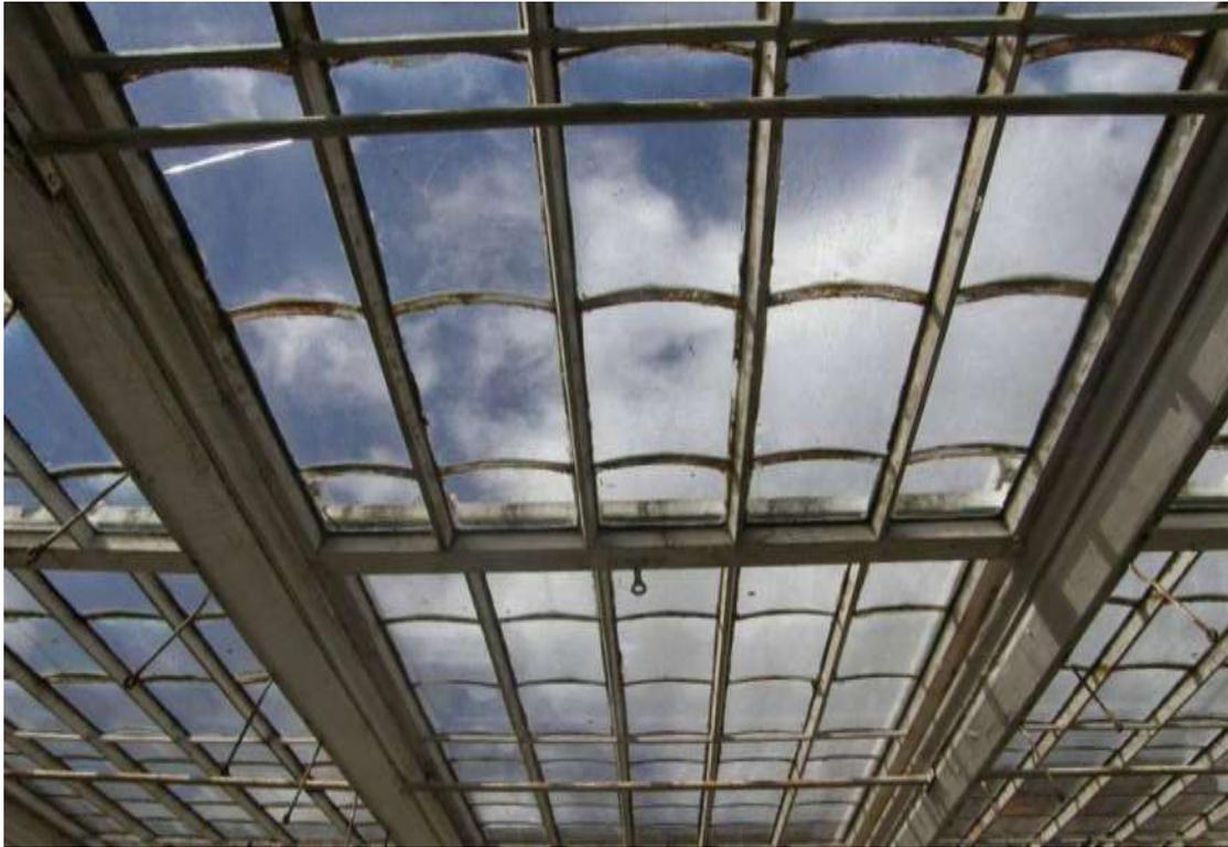
The roof of the vinery showing the lower edges of each pane of glass designed to provide better drainage
