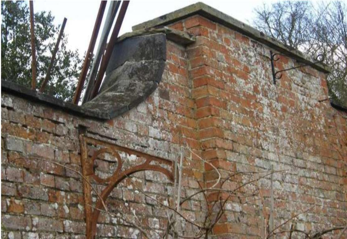
The wall bracket in the foreground is one of a series equally spaced along the West wall and the western side of the North wall. These were used to support a shelter for the plants from the intense heat of the morning sun after a frosty night
