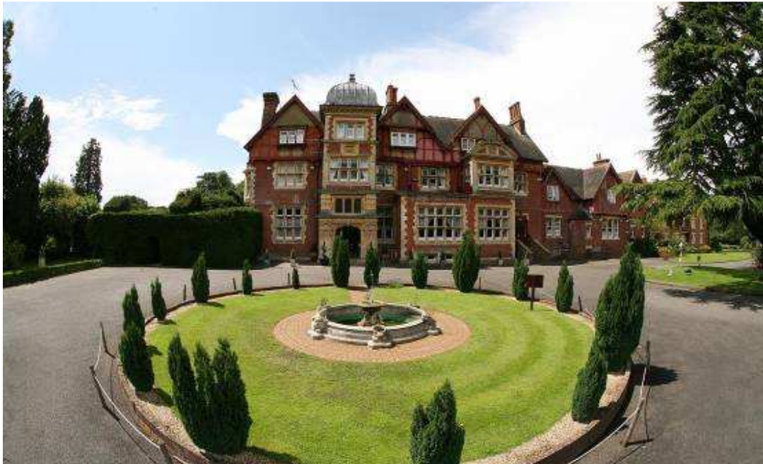
Pendley Manor, which is now a hotel
