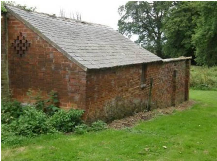
Lean-to shed taken from the outside of the WKG, situated against the southern end of the west wall. On the near wall is the diamond shaped section of brickwork for ventilation. The wall at the far end of the shed projects beyond the South wall of the WKG as it is now
