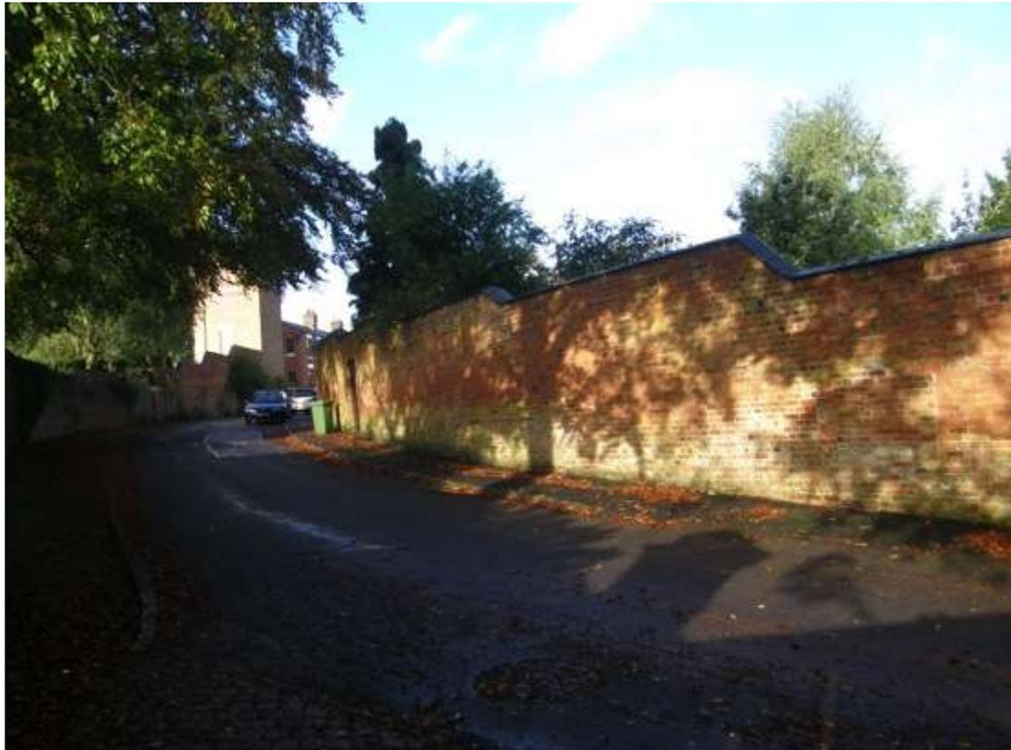
Outside of the Eastern wall of the WKG showing the steps in the top of the wall as it follows the slope of the lane. It also shows the gate that is currently used and another gate that has been bricked up. The wall of the garden around the house can also be seen on the other side of the lane with the water tower at the end.
