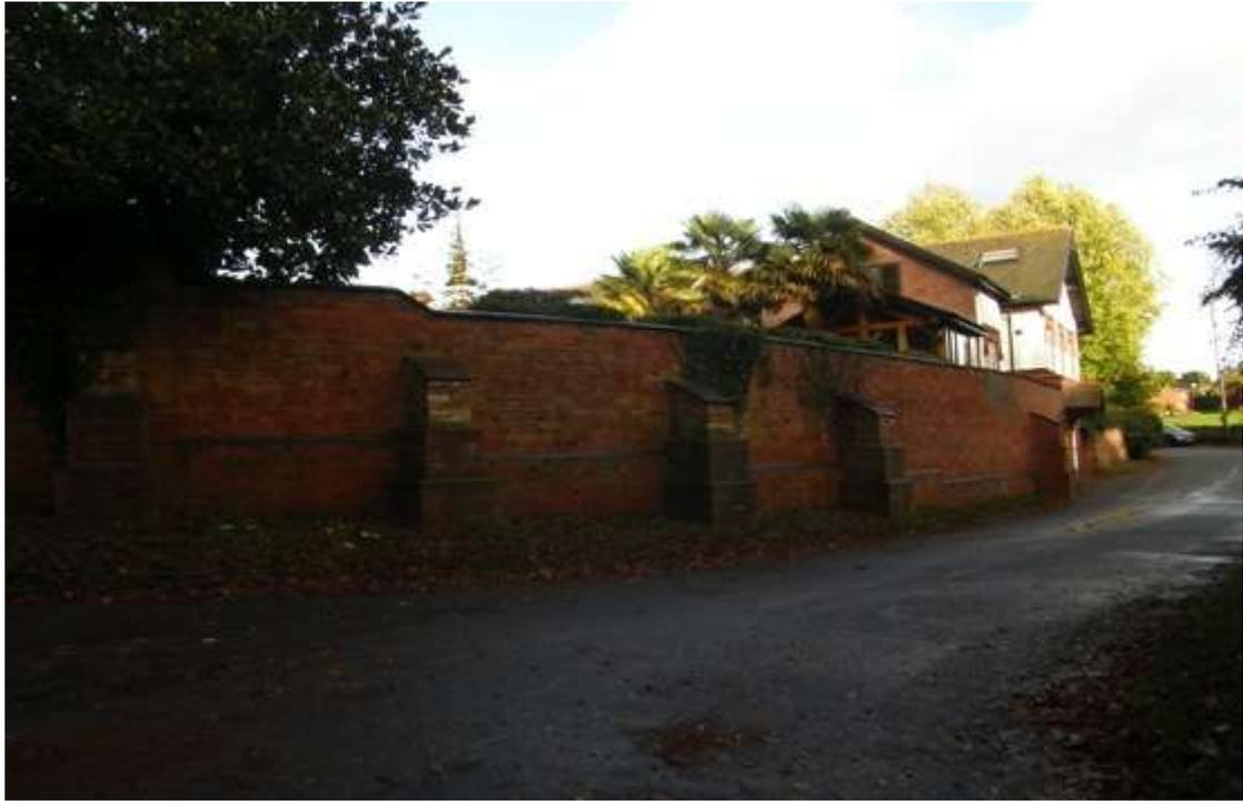
The outside of the Southern wall showing the buttresses added during development work circa 1980's to provide extra support and a stone plinth that appears as the wall follows the slope of downwards. At the end of the wall is a house and the village hall built in 1898 by Paddy Logan
