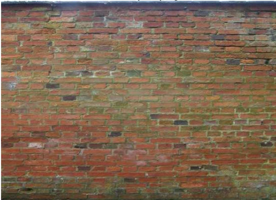
A section of the wall showing the English bond brickwork, alternating courses of headers and stretchers, capped with saddleback engineering blue bricks
