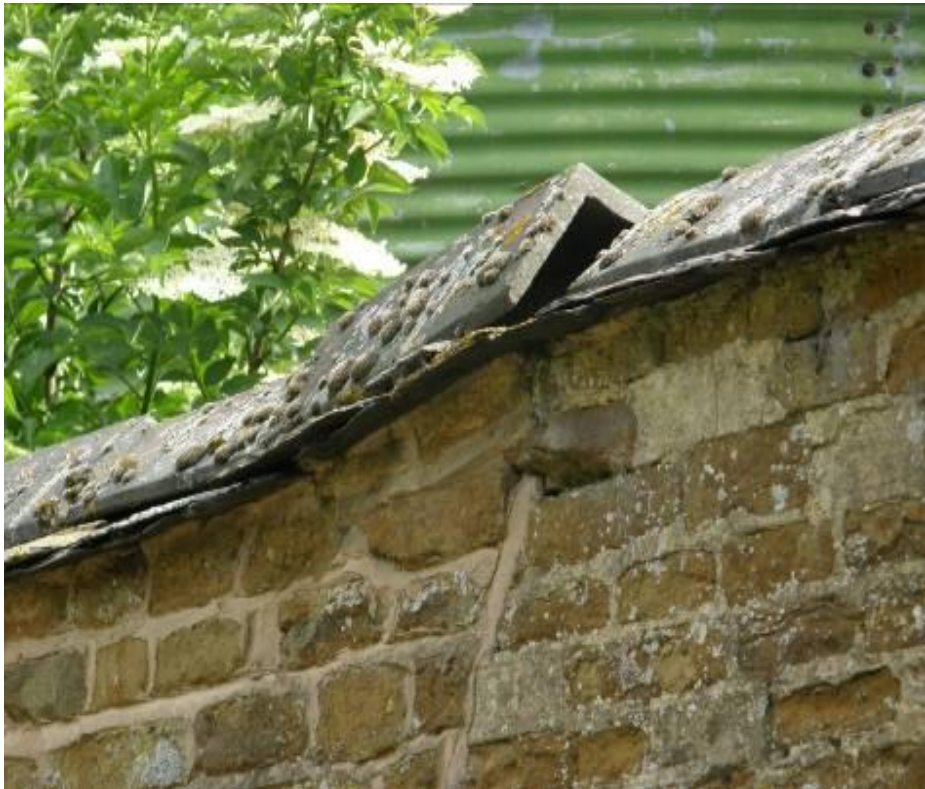
Saddleback coping and slate dripcourse
