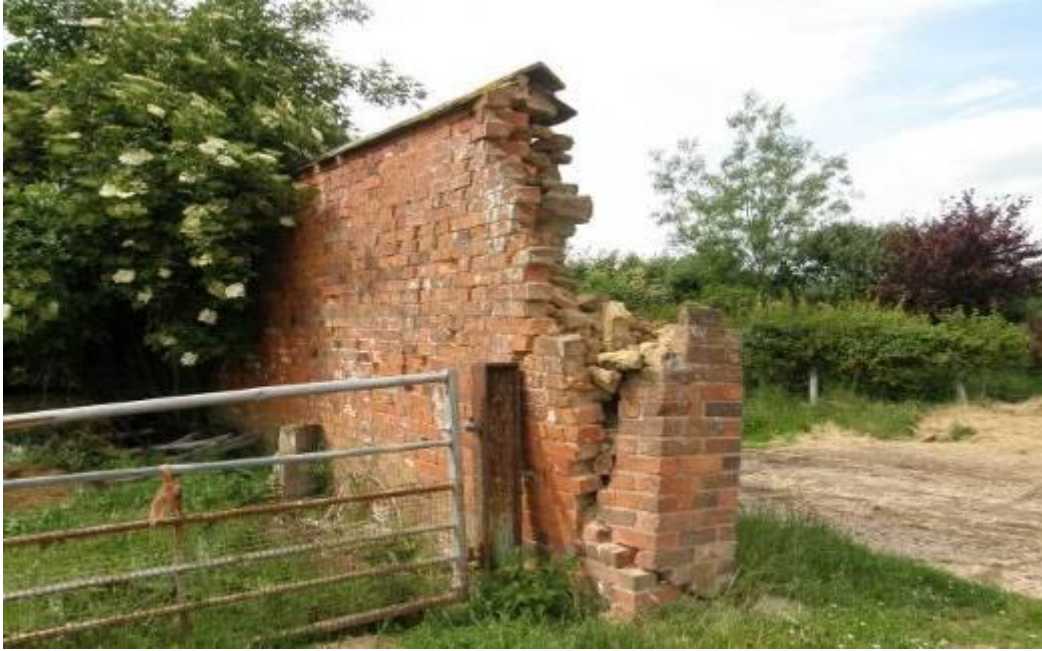
Brick lining of wall and possible gate pier
