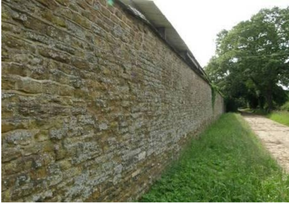
Exterior view from north of WKG ironstone wall
