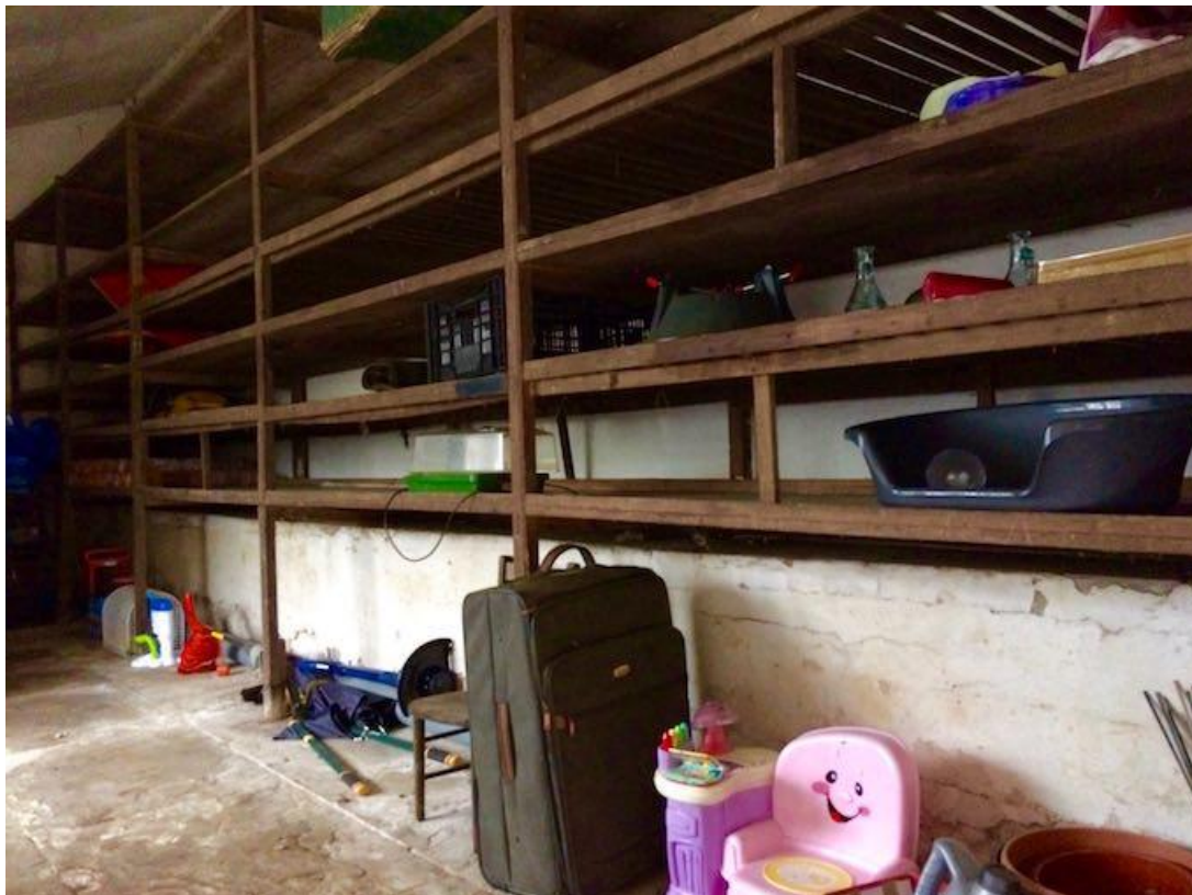
Storage racks in the fruit room – brick fire duct visible below
