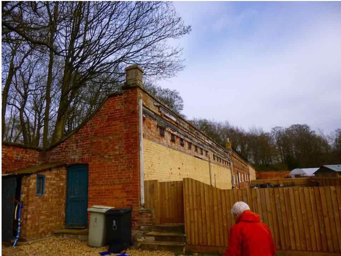
View of S facing wall with bothies behind– showing ventilator flaps
