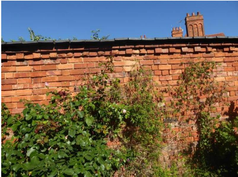
Original NE Wall of the WKG at Westbrooke House showing the brick bond, cornice and coping.
