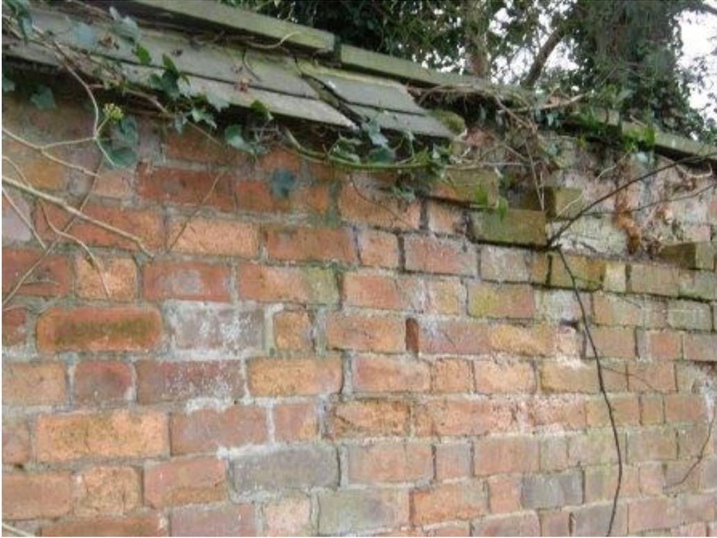
This is the outside of the north wall of section 1. This shows the double slate drip course.
