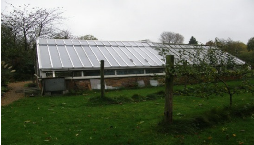
A side view of the original Messenger glasshouse built c.1879. The position of the 2 compartments is indicated by the change in the roof i.e. the replacement roof is at the door end and the original one at the far end.
