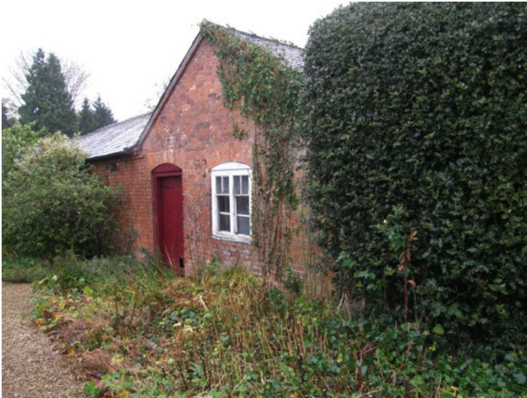
Backshed on the NE side of the WKG now used as a potting shed. Beside this the wall is replaced by a hedge
