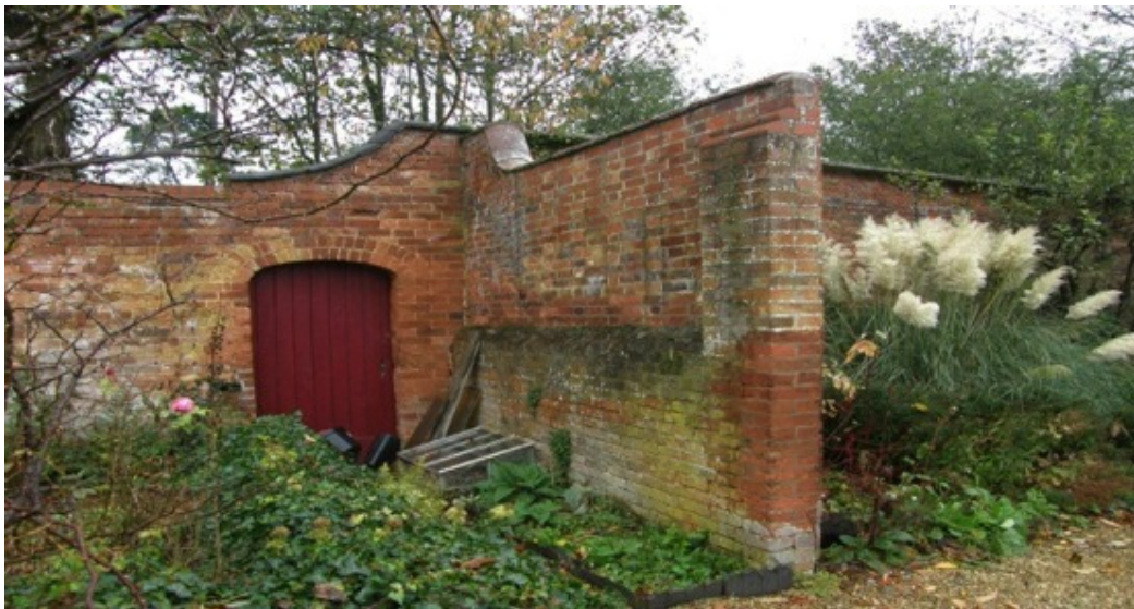
This is the projection from the NW wall that provided protection for the peach house and vinery. The door led to the boiler house situated against the wall on the outside of the garden. The glasshouse would have abutted the door and traces of whitewash can be seen on the back wall.
