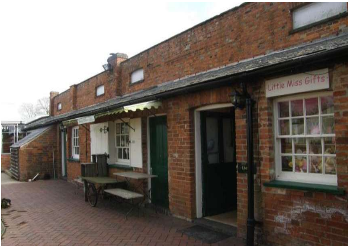
Some of the backsheds, now shops, that are behind the vinery. The lower lean-to at the end is the boiler house
