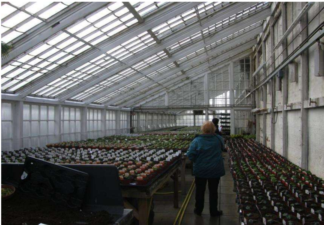
The interior of the vinery showing the central partition and weights along the back wall that are part of the original mechanism to open areas of the roof
